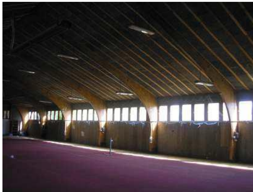
Figure 1 – Multifunctional hall built using curved poplar GLT beams in *** Hungary.
